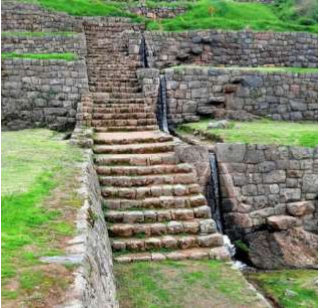
Drystone constructions – terraces – water supply in Peru
